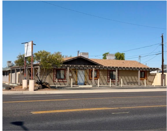
Above left: Exterior of the church building in Phoenix.
